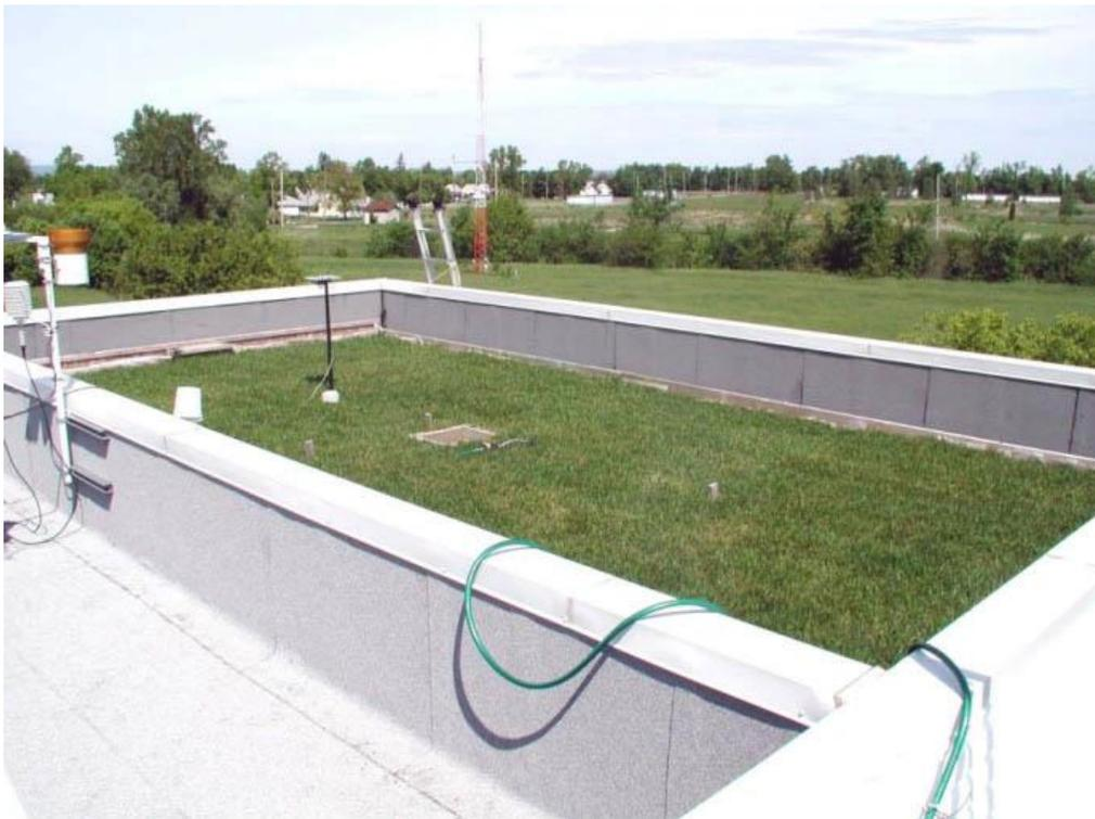
*Figure 3 Photograph of the FRF in the NRC campus in Ottawa (2002). The median divider separates the Green Roof (right) and the Reference Roof (left). The weather station is located at the median divider. (Liu, 2003)*
